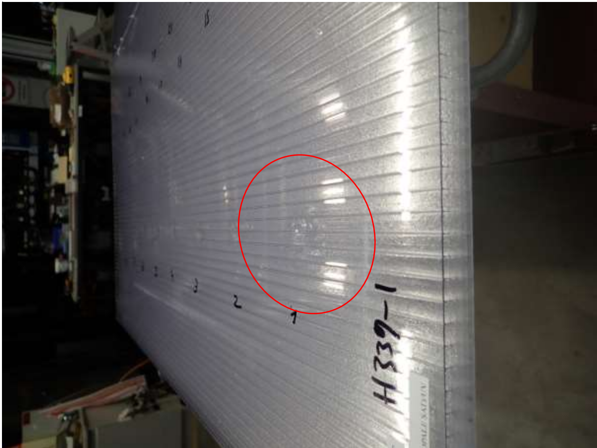
Figure 7: Visible dent and a surface deformation and an internal material defect visible (shot with a diameter of 50 mm)
